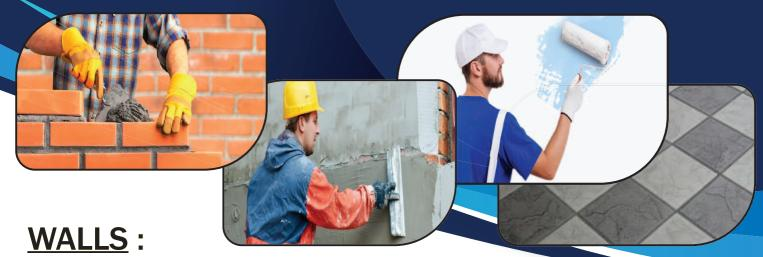
Outer walls are 9" and inner wall are 6" thickness red/flyash brick, withcement mortar (1:4 prop).
