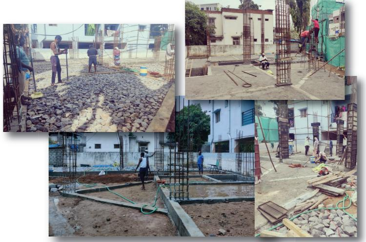
They are backfilling the areas inside the plinth beams constructed on top of the foundation with the soil extracted during excavation and/or other material for Constructing I.B MALL
